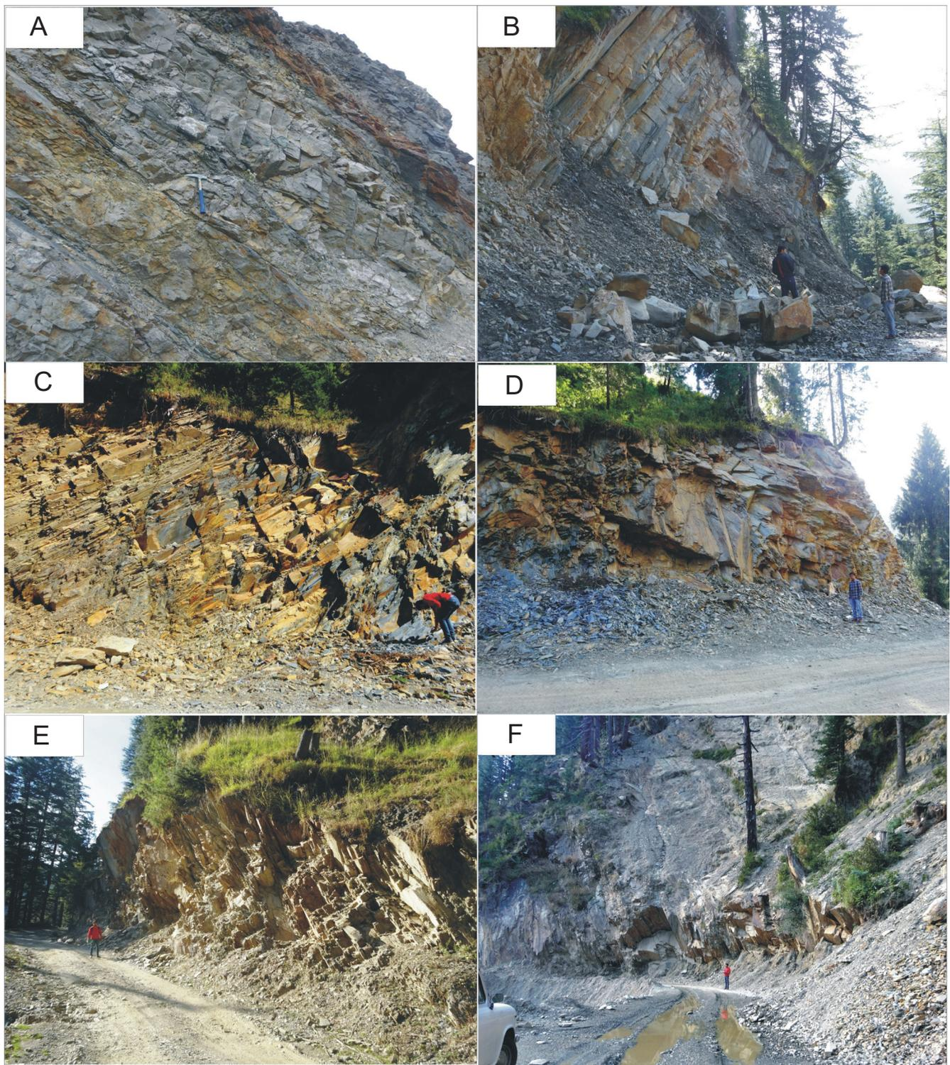
Fig. 2—Field photographs showing vulnerable rock slopes, (A) Slope face showing failure due to intersection of bedding plane and joint set (B) Large block of rock failures (C) Closely spaced joint in phyllitic rock (D) Wedge failure in highly fractured rock mass (E) Rock slope showing highly blocky structure (F) Slope face showing wedge failure due to intersection of joints.
